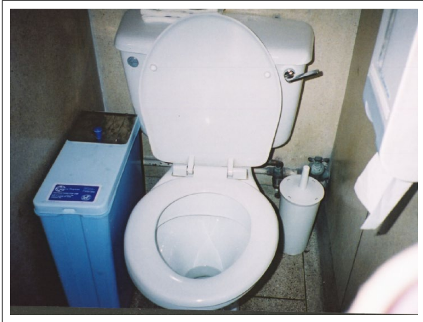
Figure 3. Inside a cubicle in the Ladies. © author.
